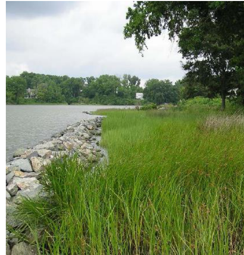
Typical Sill Living shoreline engineering guidelines New Jersey Department of Environmental Protection, 2016
