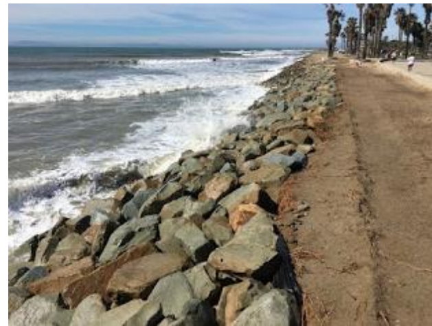
Revetment Ventura rock revetment, Ventura river ecosystem, 2017
