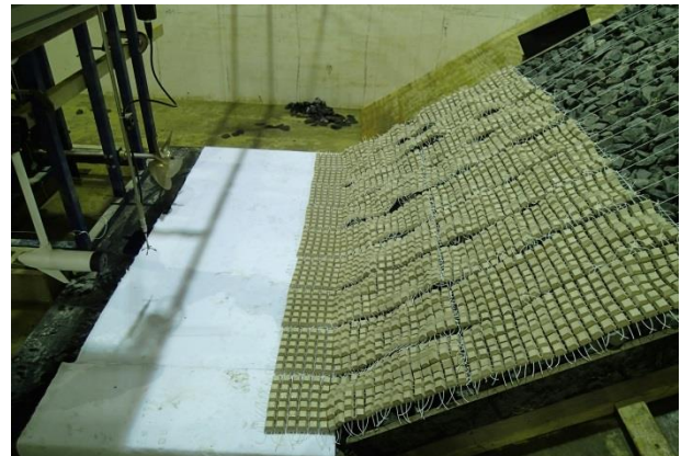
Figure 1 - ACMs in place over the rock slope during the Handysize vessel tests.
