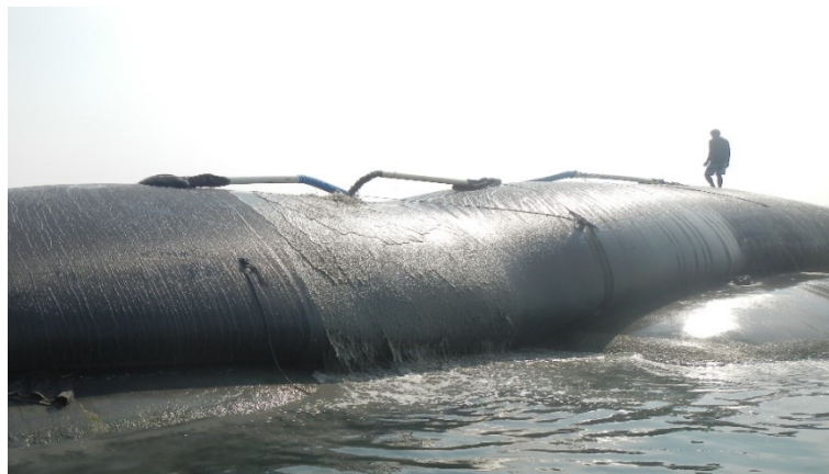
Figure 12. Installation of Geotextile Tube as a core of Breakwater
