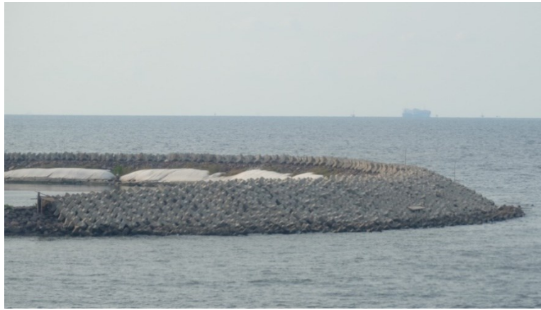
Figure 13. Breakwater with Geotextile Tube as a core
