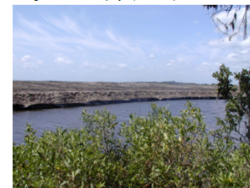
Levee Reach J-1 Construction
