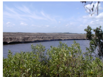
Levee Reach J-1 Construction
