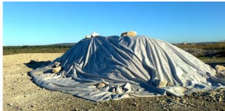
Preservation of the petty surge by nurseryman during the work period
