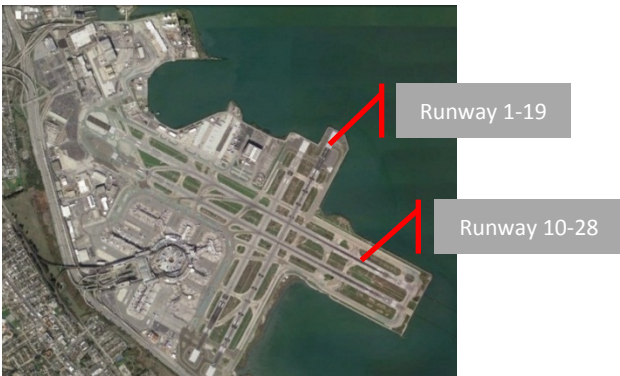
Figure 1 - SFIA Shoreline and Runways
