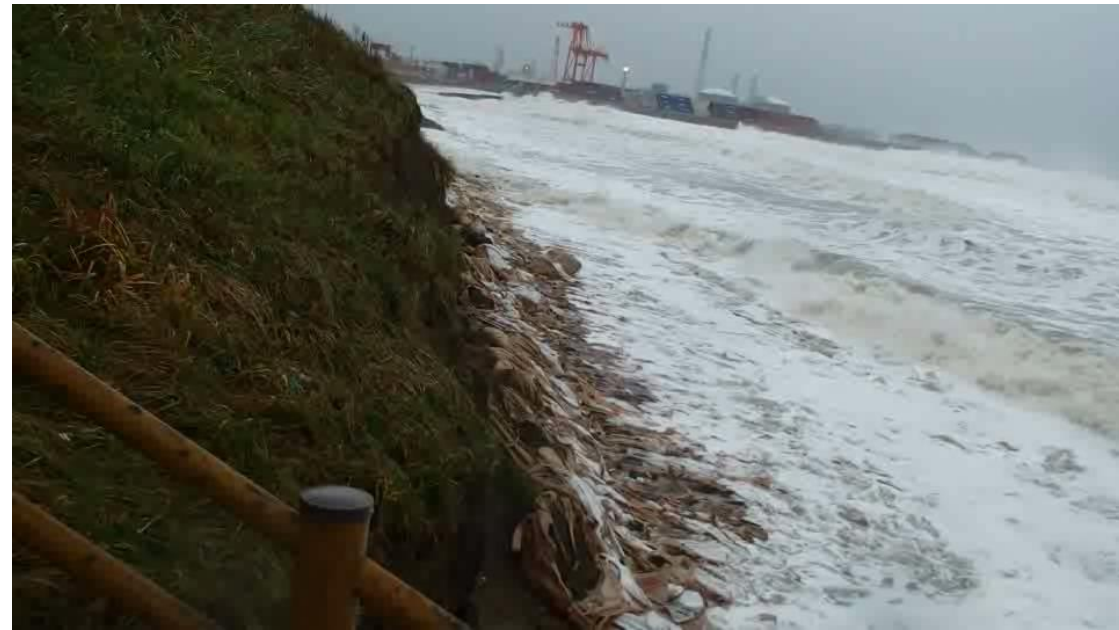
Erosion of embankment toe by the waves
