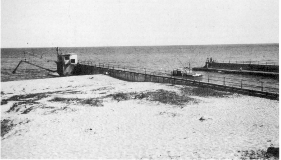
Fig. 3. Pumping plant near outer end of north jetty.
