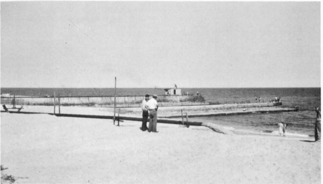
Fig. 4. Discharge line south of south jetty.
