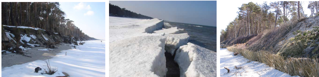
Figure 3. Beach at CRS Lubiatowo: dune erosion after heavy storm, photo: G. Różyński (left), ice barrier preventing further dune erosion, photo: G. Różyński (middle), rehabilitation of dunes with stick fences in spring, photo D. Piotrowska (right).
