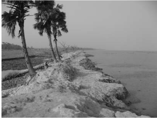
Figure 3: River bank erosion in Southkhari.
