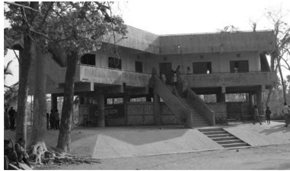
Figure 4: Cyclone shelter in Southkhari.
