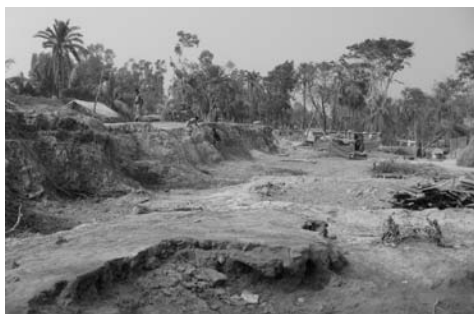
Figure 6: River shore erosion in Sombonia.
