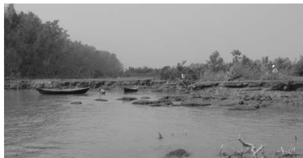
Figure 7: Erosion behind bank in Sombonia.
