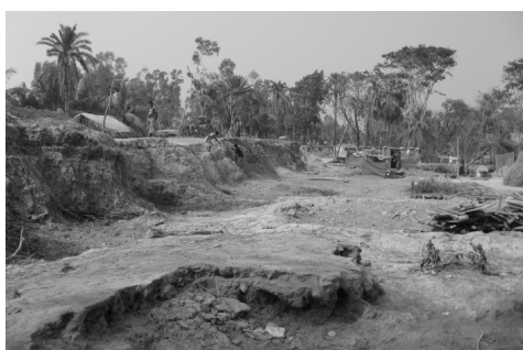
Figure 6: River shore erosion in Sombonia.
