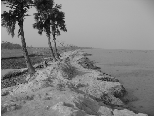
Figure 3: River bank erosion in Southkhari.
