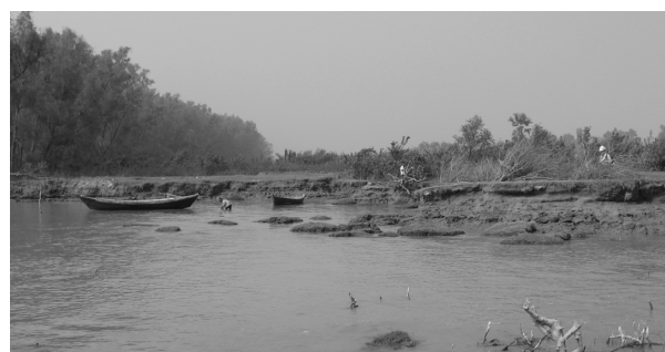
Figure 7: Erosion behind bank in Sombonia.
