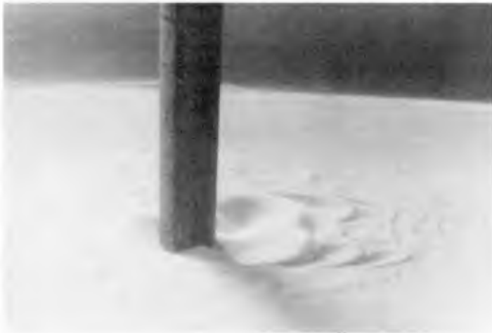
Figure 6. Initial stages of scour development.
