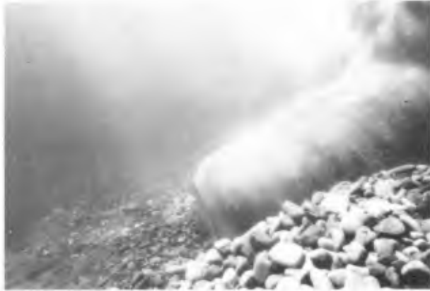
Picture 1 Underwater picture taken at the offshore foot of No.17 detached breakwater (1).
