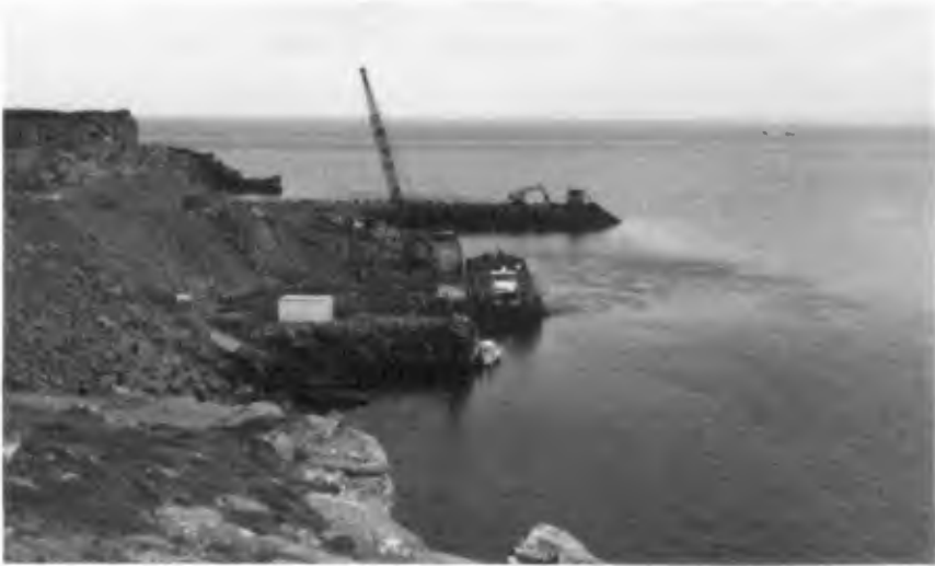
Figure 2 Quarry Operation Adjacent to Breakwater Construction
