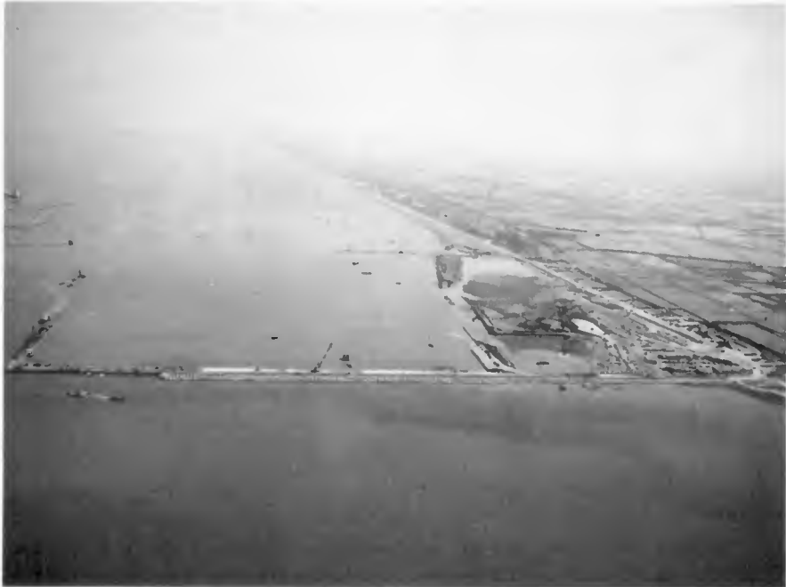
Photo 1. Aerophoto of Hsin-Ta LNG Terminal (under construction)
