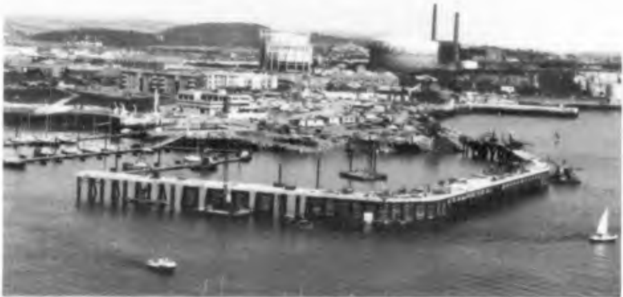
Figure 10: Marina Nearing Completion
