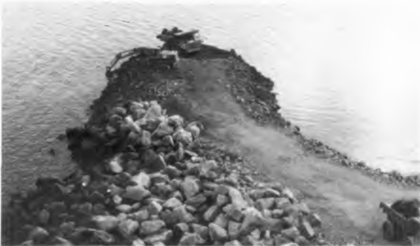
Figure 3 Breakwater Construction
