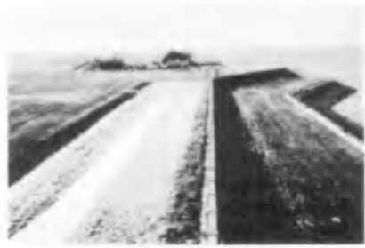
Fig. 4 Eastern Scheldt dike (with return wall)
