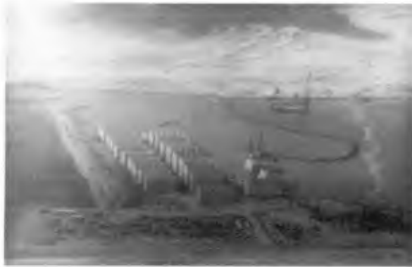
Figure 3. Caissons made on the beach where is dredged for harbor basin later
