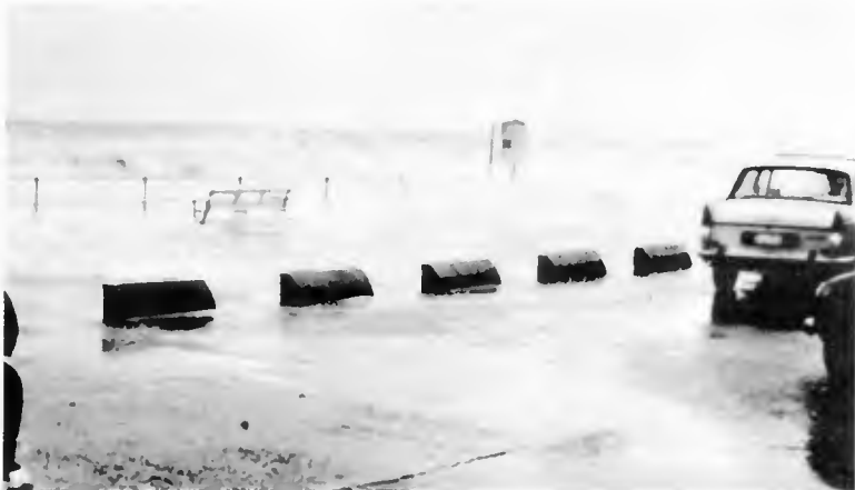
Picture 2 : During storms, waves overtop the existing sea-dike (winter 1975)
