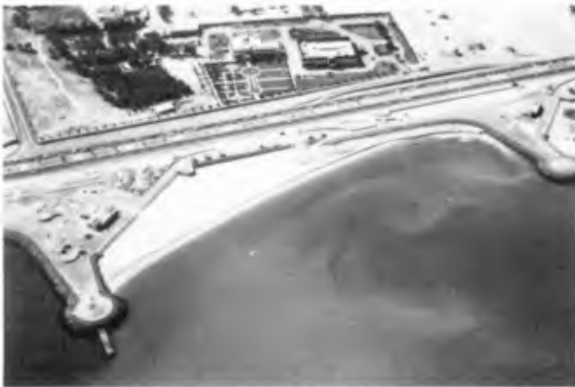
FIGURE 4. (a) Typical pocket beach designed for the KWF project. Alignment is into the predominant wave direction to minimize longshore sand losses. Retaining structures double as promenades and outfalls. (b) Pocket beach nearing completion on 12 December 1985 along the KWF project.
