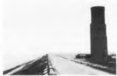
Fig. 6 Eastern Scheldt dike with return wall and roads behind the crest
