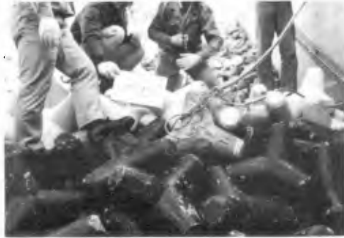
Photo 3 The Condition during Placement
