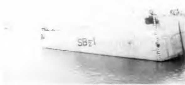
Figure 6. Caisson slides toward water under process of Slide-to-Float method
