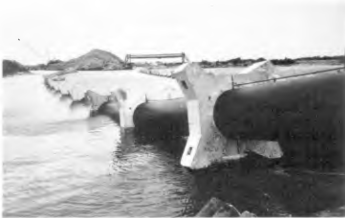
Figure 1: Typical star weights, Richards Bay HDPE pipeline
