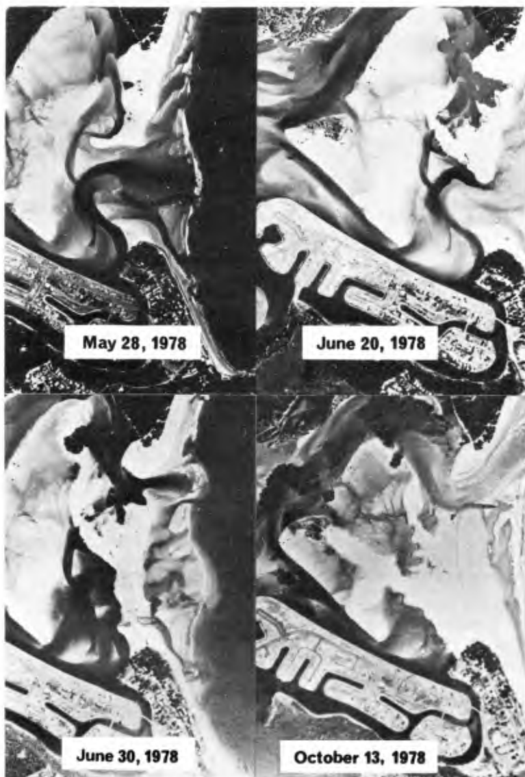
FIGURE 5 - Photographs showing progress of the works
