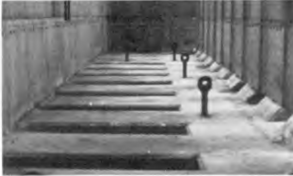
Fig. 18.- Lower Part of Wave Chamber of the Seawall
