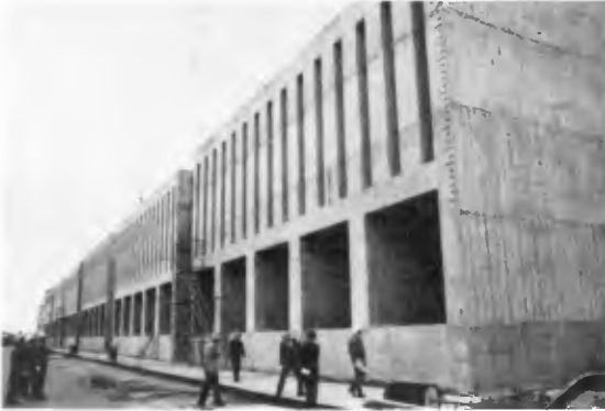
Fig. 16.- Completed Caisson for Seawall
