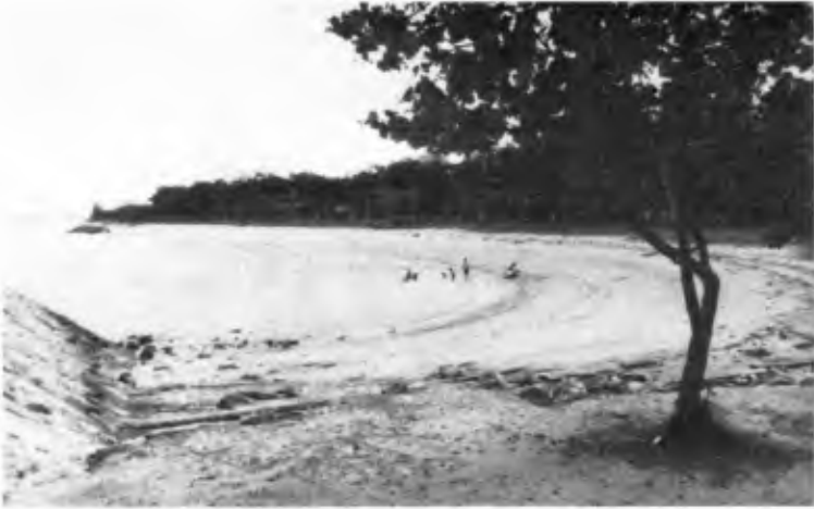
Plate 1. Typical J-shaped bay between headland breakwaters (Phase I reclamation).
