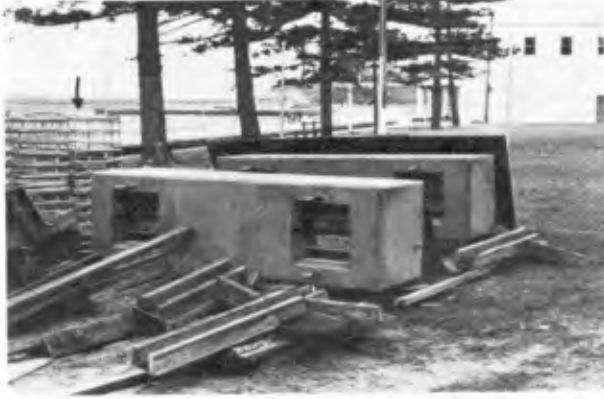
FIGURE 7 PRECAST REINFORCED CONCRETE HEADSTOCKS
