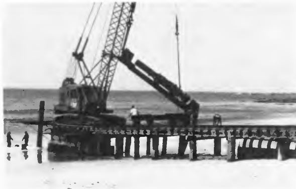
FIGURE 4 PILE DRIVER BEING LIFTED INTO POSITION
