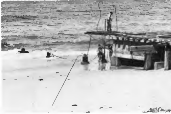
FIGURE 5 JACKETS BEING JETTED IN AROUND PILES
