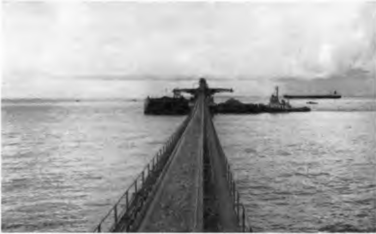
Plate 3. Loading of fill material from the belt conveyor onto barges.
