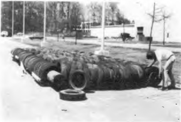
Plate 2. Assembly of PT-Breakwater.
