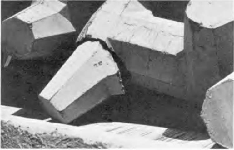
a. Typical fluke breakage
