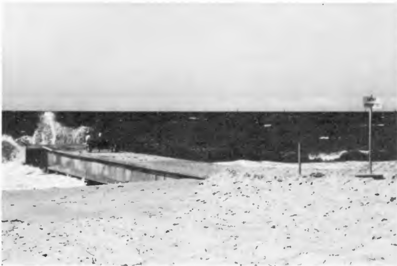
FIGURE 14 WAVE IMPACTING ON OUTLET UNIT
