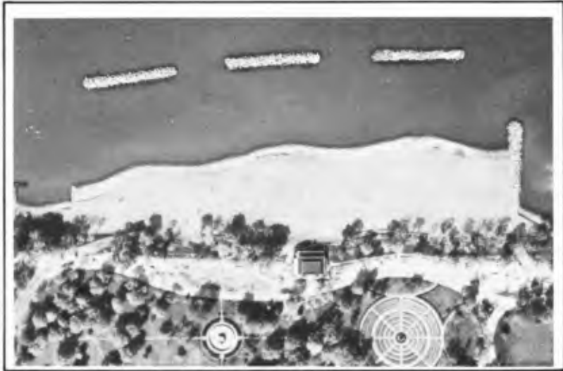
PHOTO 1: IMMEDIATELY AFTER CONSTRUCTION, OCTOBER, 1977
