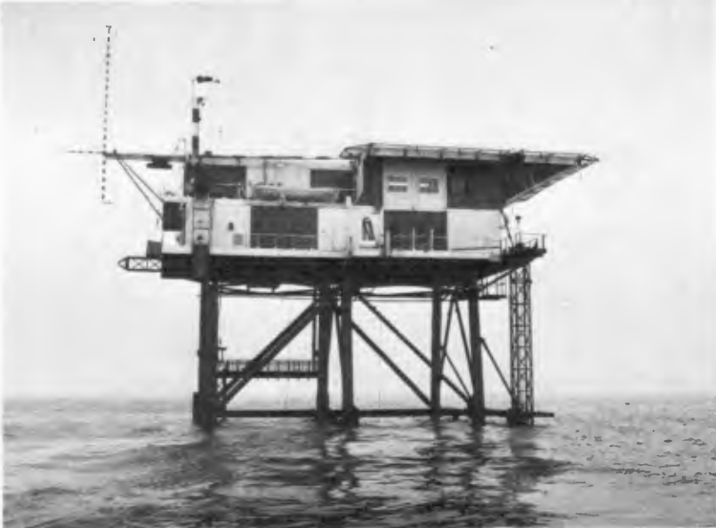
Figure 2: side-view of MPN (north-side)
