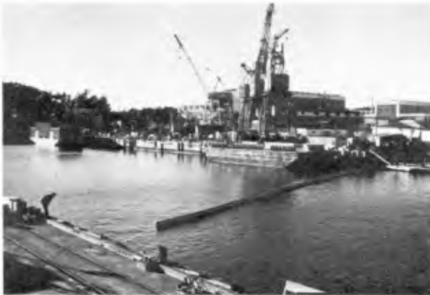
Figure 15 The curtain in the closed and anchored configuration as seen looking into the Pier 20-21 berth
