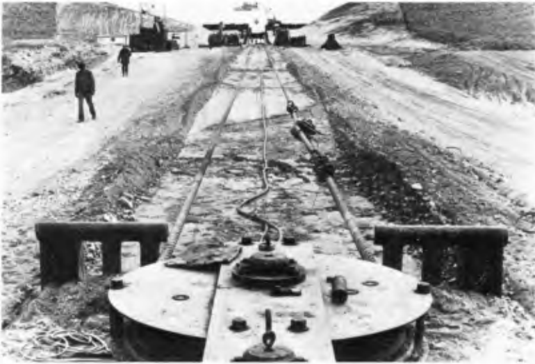
Photo 1. Pipeline Pulling of the Flags Gasline at St. Fergus.
