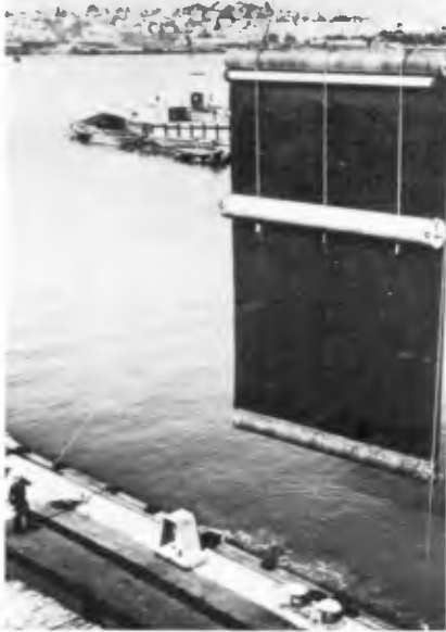
Figure 11 Rigging a curtain section for proper buoyancy
