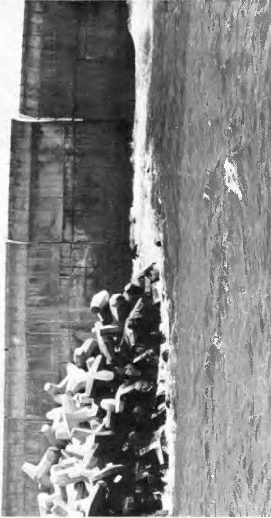
Figure 2 Dolos removed from the front of the seawall and broken dolos and superstructure (photo from GAS)
