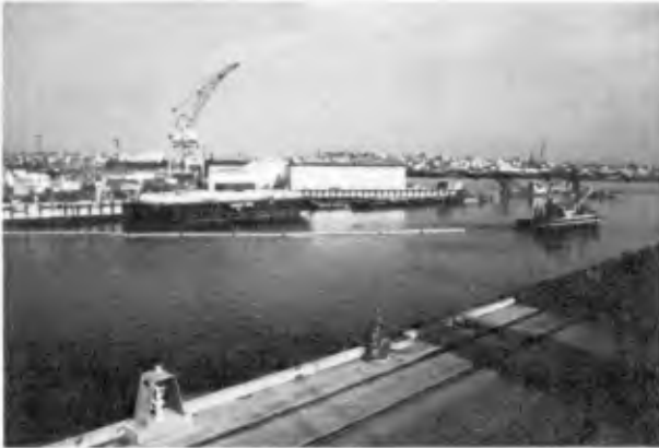
Figure 14 The curtain being opened by the Sea Mule yard tug
