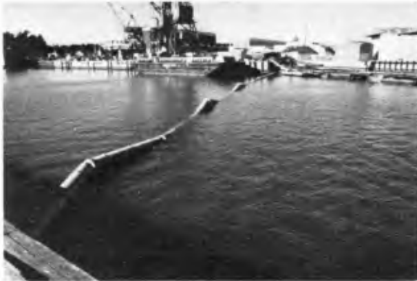
Figure 13 Surface buoys while raising anchored sections from the mud during a rising tide
