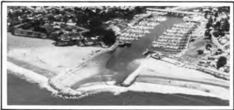
PHOTO 1: SANTA CRUZ HARBOR IN SHOALED CONDITION
