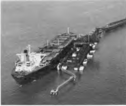
Offshore loading facilities at Hay Point, Queensland
