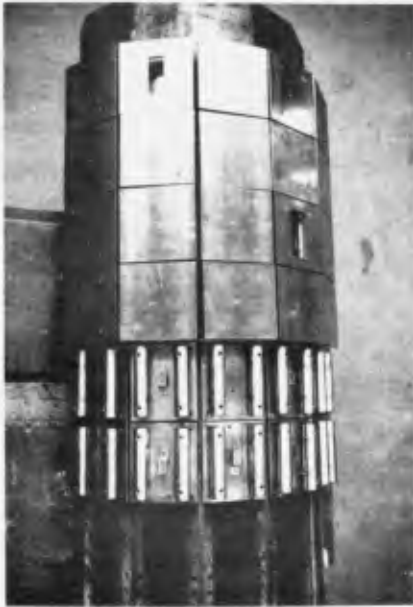
FIG. 4 SHIELD WITH 50 PRESSURE CELLS
