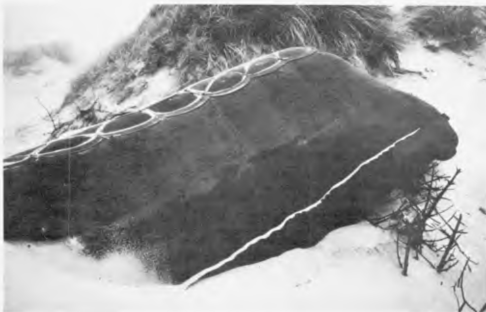
Fig. 3. Tubes wrapped into a filter sheet.
