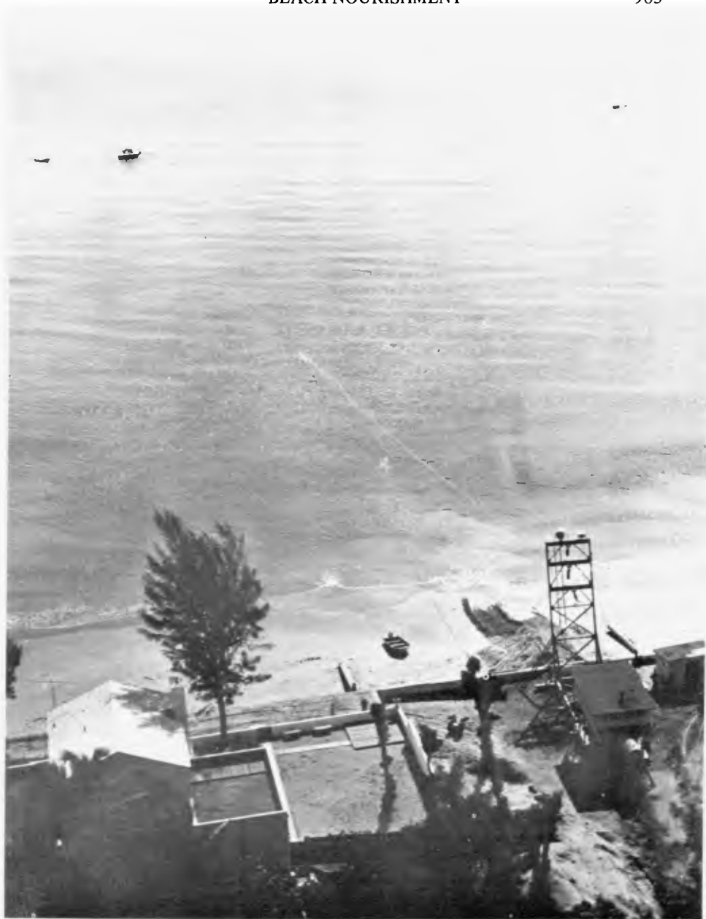
Photograph 4. Aerial View of Drag Scraper
