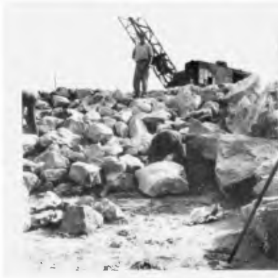
Fig. 18 - Detail of the construction of groyne in Cova do Vapor
