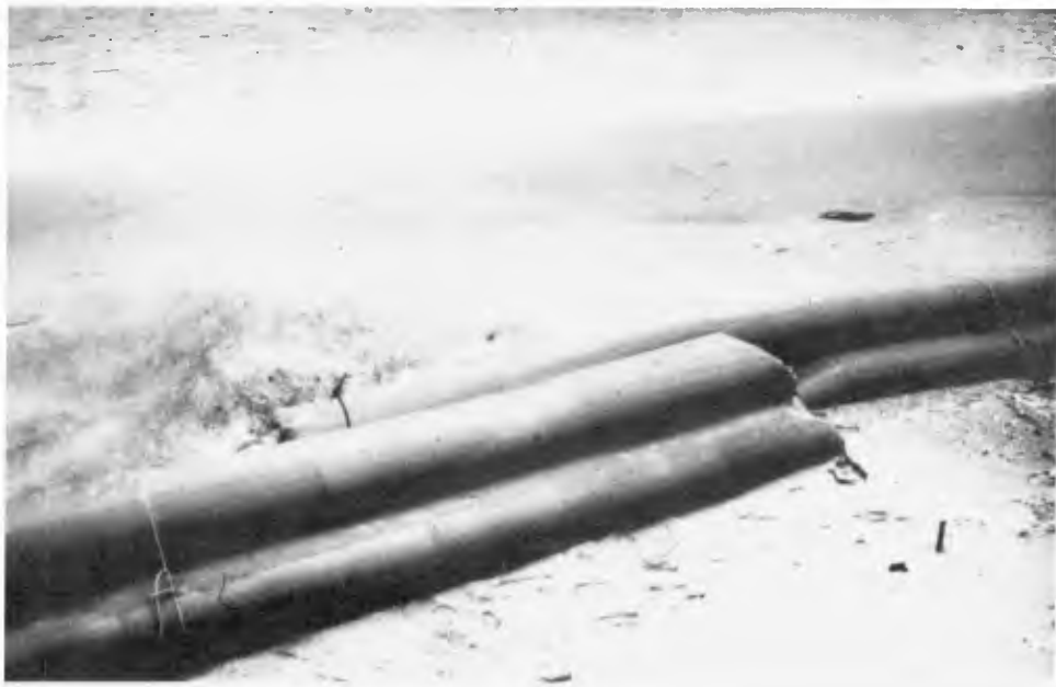
Fig. 2. Structures composed of sand tubes with diameter 0.7 m (1 tube on top of 2)
