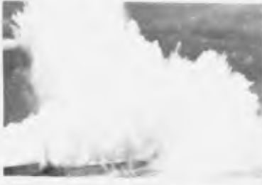
FIG. 17. - LARGE WAVE OVERTOPPINGS AT SEA-WALLS OF WAKAYAMA HARBOR
