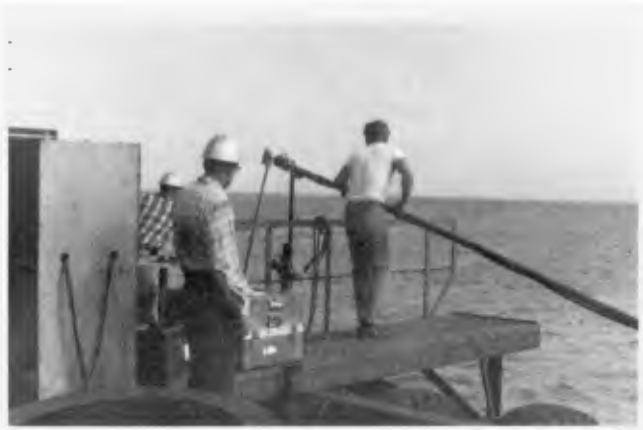
FIG. 5. - INSTALLING METER AT SAN NICOLAS PIER
