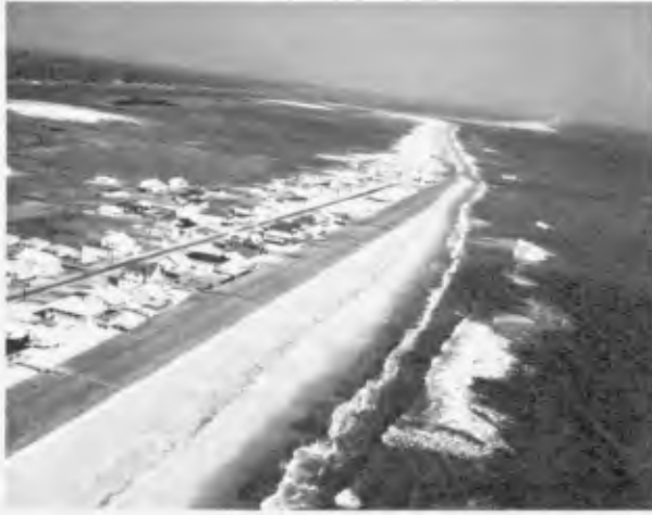
PHOTOGRAPH 1 - VIEW NORTHWARD OVER CAROLINA BEACH PROJECT IN 1965. NOTE CHANGE OF SHORE ALIGNMENT CENTER BACKGROUND OF PHOTOGRAPH.
