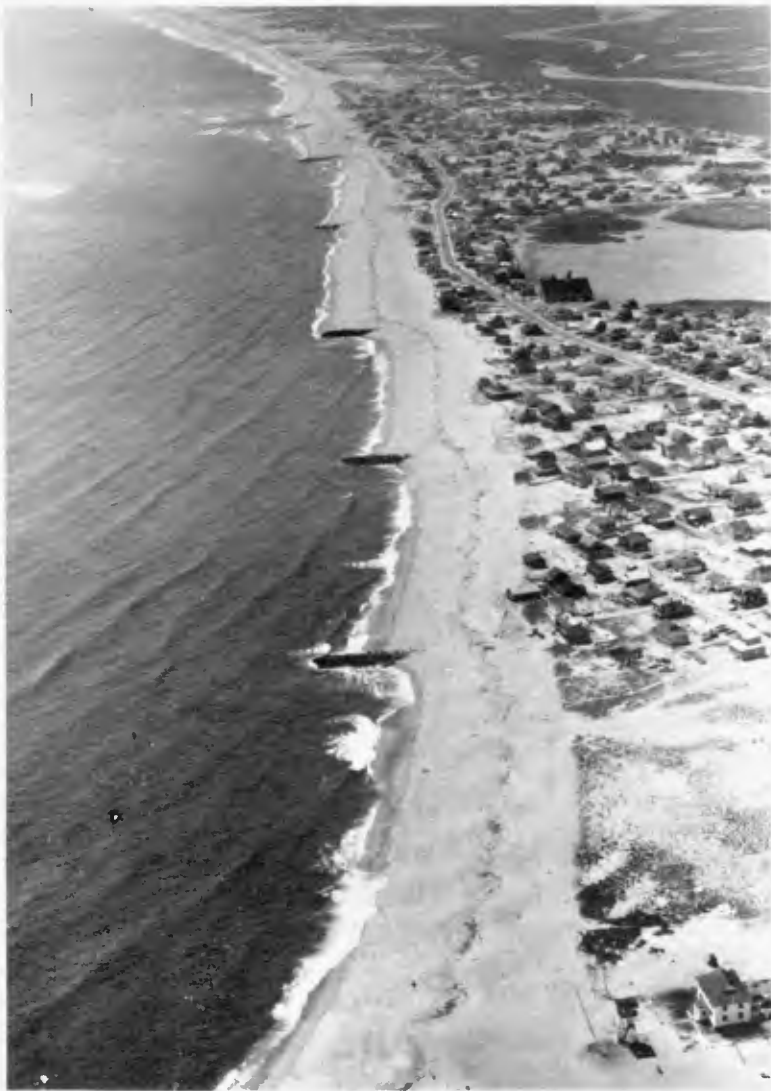
Fig. 2 View looking south along the Plum Island beach, Massachusetts, just south of the Merrimack inlet. Coast Guard station in foreground is located on the wave refraction diagram of Figure 1. Note accumulation of sand on the south side of the groins and the oblique approach of the wave crests from the southeast. The groin field is located inside the ebb-tidal delta and is in an area of local reversal of longshore drift which results from wave refraction around the ebb-tidal delta (Fig. 1). In the far background of the photograph, drift resumes its normal southerly trend. Photograph taken June 1968.
