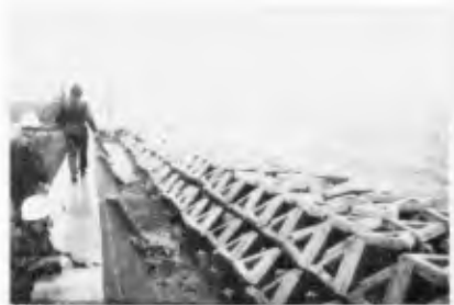
FIG. 23. - SEA-WALL OF THE KANSAI E. P. CO. LTD. DURING A TYPHOON, 1961
