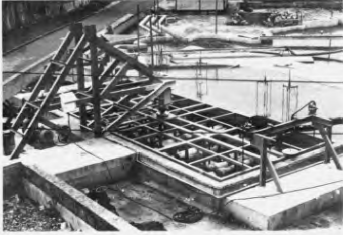
Fig.2 PLUNGER OF THE TSUNAMI GENERATOR
