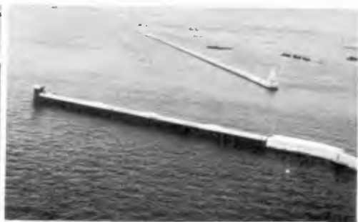
Fig. 39. Steel-pipe breakwater after completion.
