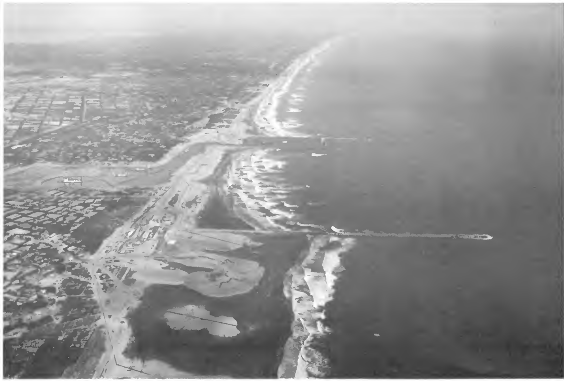
Kashima Industrial Area
