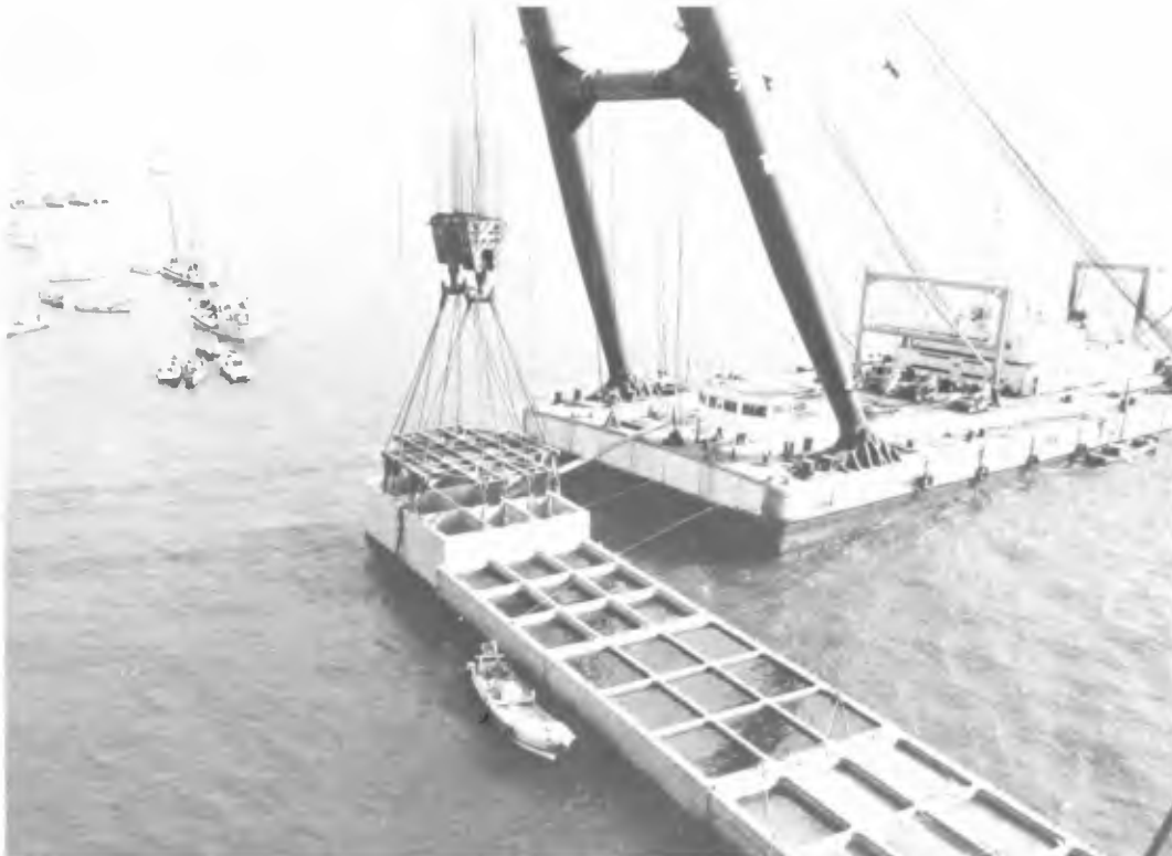
Kobe Harbor Breakwater
