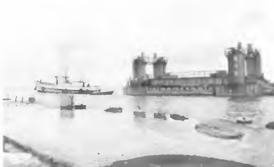
Fig. 6. Tugging a caisson with the aid of floats.
