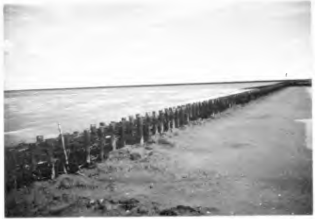
Fig. 10. Main dam with brushwood groyne (early stage).
