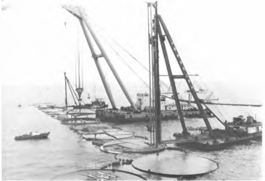
Kobe Harbor Quaywall
