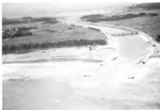
Fig. 8. Mouth of Simbori River diversion channel.
