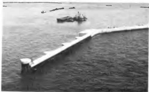
Fig. 38. Steel-pipe breakwater after completion.
