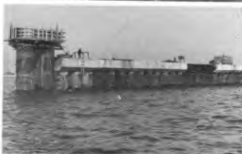
Fig. 36. Steel-pipe breakwater in near completion in the Port of Osaka.
