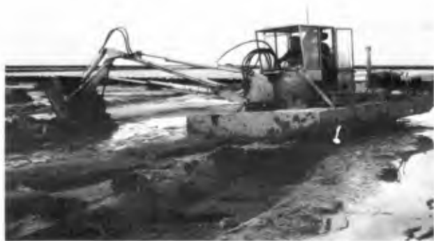
Fig. 13. Mechanization "Floating" excavator in low sedimentation field.
