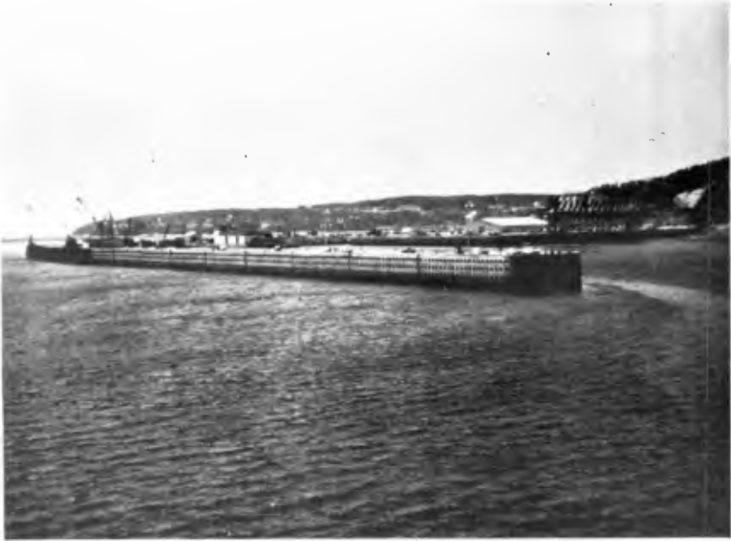
Fig. 6. Baie Comeau harbor breakwater (National Research Council of Canada).
