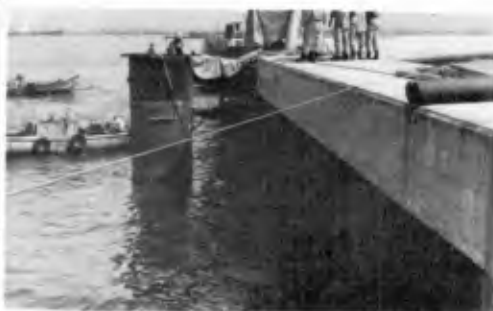
Fig. 37. Steel-pipe breakwater undergoing horizontal load tests.
