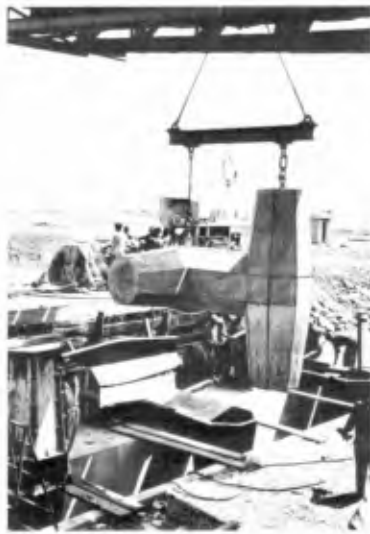
Fig. 2. Lifting a 19-3/4-ton Dolos from its mould.
