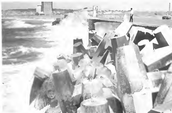
Fig. 4. Difference in run-up and splashing between rectangular blocks (background) and Dolosse (foreground).
