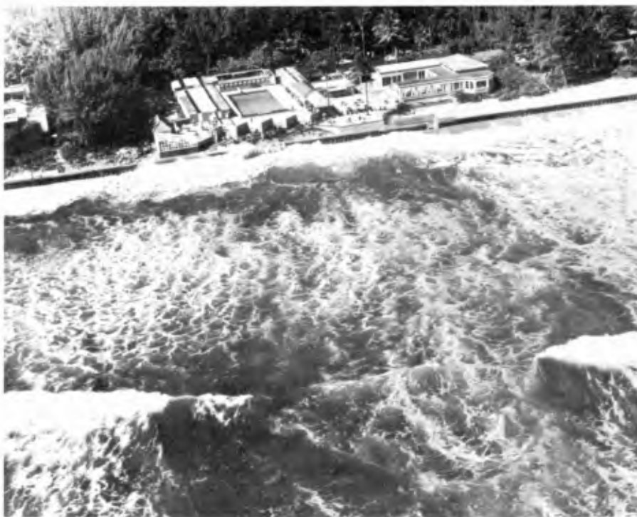
FIG. 10. WAVE ACTION ON VERTICAL (STEEL SHEET PILE) WALL, JUPITER ISLAND, FLA.
