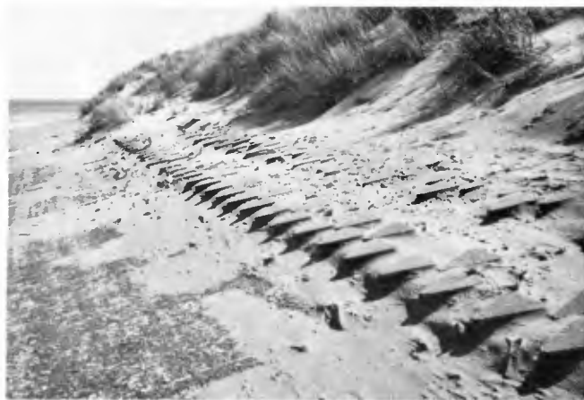
FIG. 8. SAND DEPOSITS ON REVETMENT OF FIG. 7 (TEXEL)
