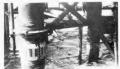
D BOLTED JOINT E HOSES FOR CARRYING ELECTRICAL WIRES
