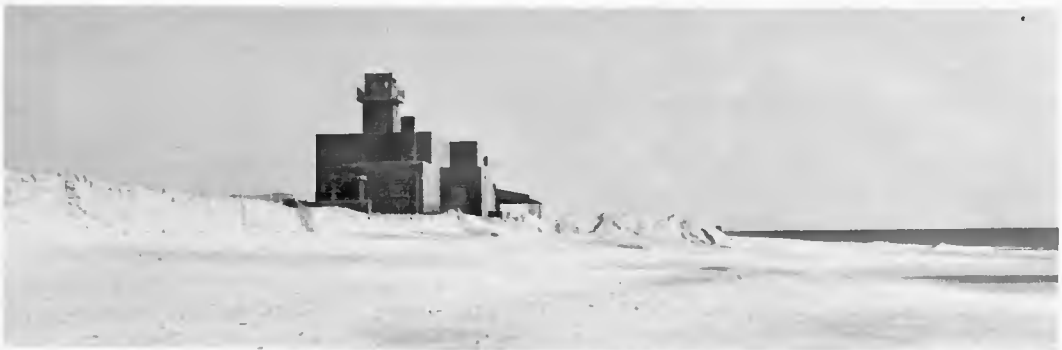
Fig. 7. Erosion at Gilgo State Park pavilion, early 1960.
