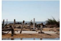
Figure 1 - House pushed over by flood loads during Hurricane Ike. The failure occurred at the connection level between the floor beam and the piles (FEMA 2009).
