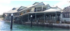
Figure 4 - Swansea Channel foreshore building collapse due to bed scour (Photo: 8/2/2016 Fire & Rescue NSW).
