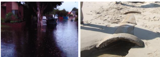
Figure 2 - Back street flooding caused by blocked drains
