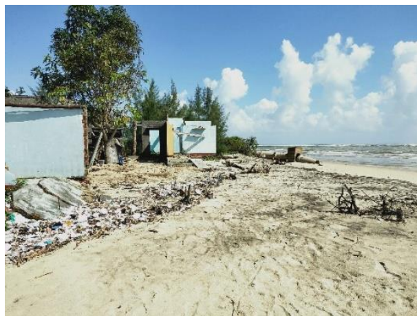
Figure 2. Eroding beach causing damages to properties and infrastructure
