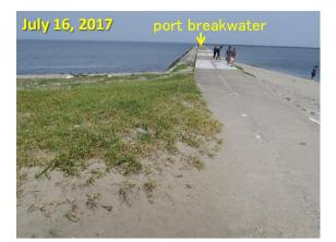
Figure 7. Sand deposition along east end of west beach and over port breakwater.
