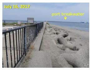
Figure 8. Sand deposition on slope along eastern edge of port breakwater.
