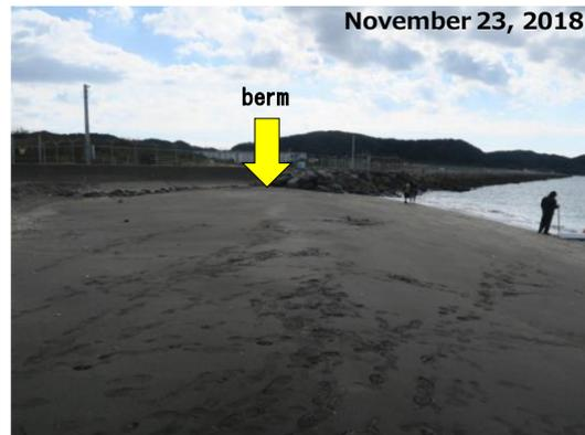
Figure 6. Shoreline obliquely intersected with seawall and a high berm (St. A).
