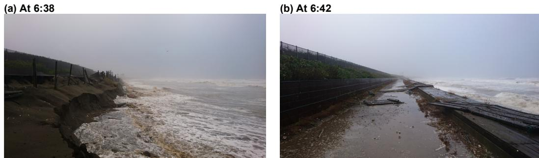
Figure 4. Erosion of sand mound along the coastline and wave overtopping to walkway in Hishinuma area during T1721 measured at 6:38 and 6:42 on October 23, 2017, respectively.
