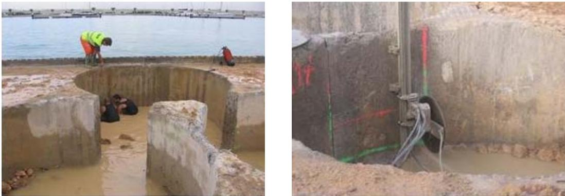
Figure 1.- Construction of wave-dissipating chambers, (a) circular cells and (b) diamond wire cut.
