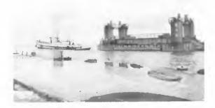
Fig. 6. Tugging a caisson with the aid of floats.
