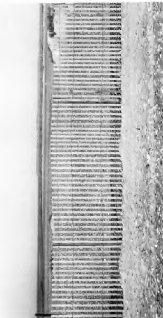
FIGURE 4. SLAT-TYPE SAND FENCING
