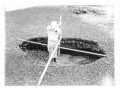
Photo 1(a) A large hole formed behind a seawall.
