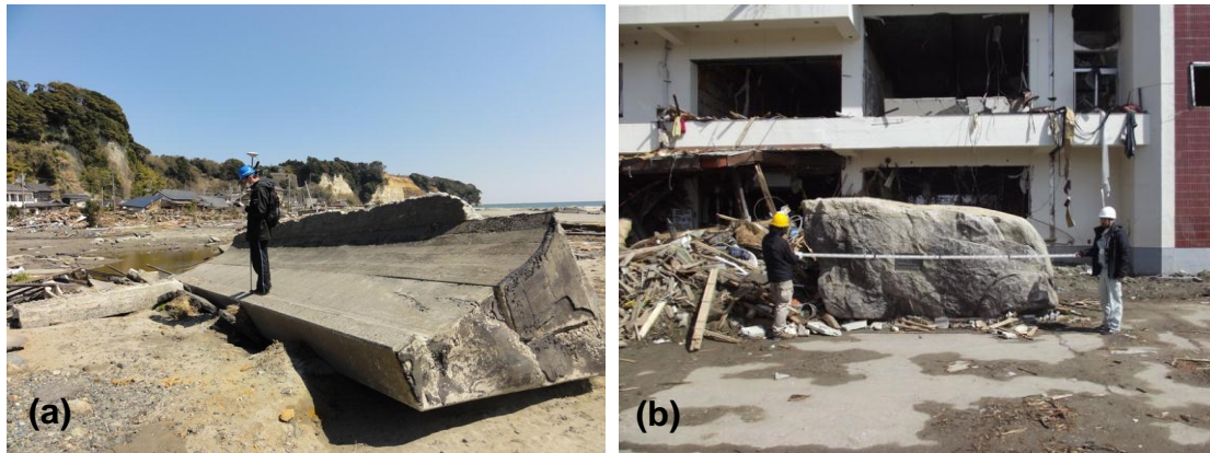
Figure 1. Relocated tsunami boulders observed in the 2011 Tohoku earthquake tsunami field survey. (a) A relocated concrete seawall block (0.5x1.6x2.24x10 m in size with an estimated weight about 56 ton) in Nakoso, Fukushima Prefecture (Sato et al., 2012). (b) An overturned boulder sitting in front of the city arena (2.0x2.1x3.6 m in size with an estimated weight about 38 ton) in Rikuzentakata, Iwate Prefecture. (Liu et al., 2013)
