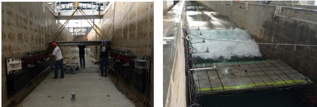
Figure 4. Installation of the bridge specimen on the bent caps (left) and turbulent bore slightly before impacting the bridge specimen (right)
