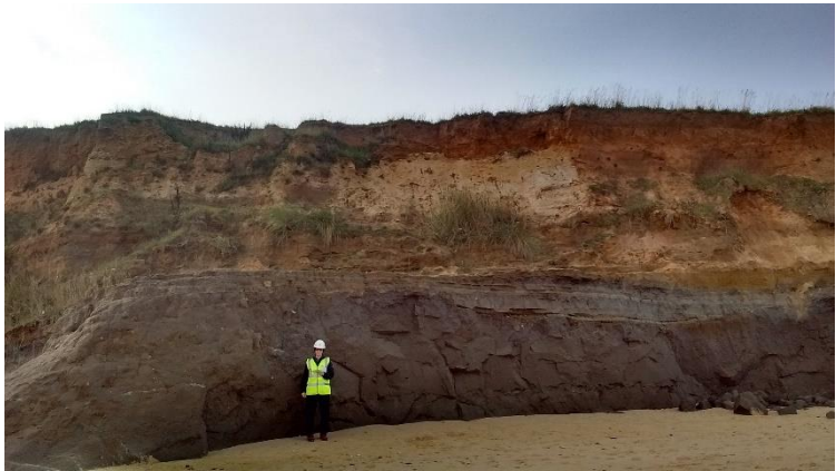
1993 a line of defence section was removed after failure leaving the soft cliff unprotected
