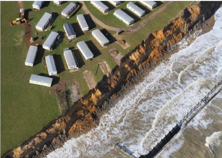
1960s line of defence was designed to reduce cliff erosion rather than entirely prevent it
