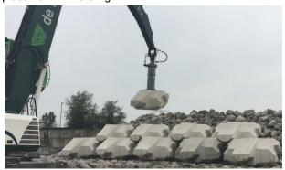
Figure 4: Placement of 6.5ton XblocPlus
