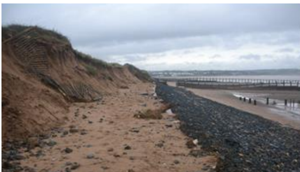
Figure 3. Dunes and beach before scheme (gabions on lower dune face).
