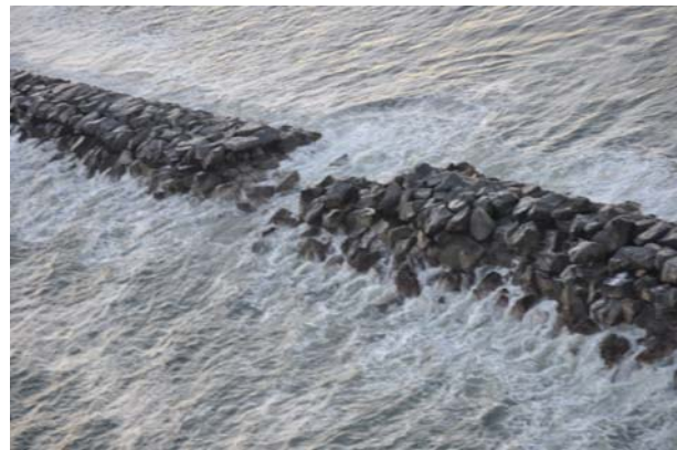
Figure 1. Breakwater Damage
