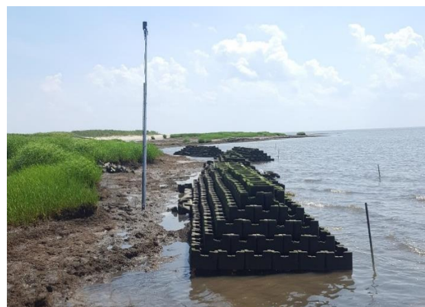
Figure 2 - Living shoreline breakwater structure exposed near low tide at Gandy’s Beach, NJ.
