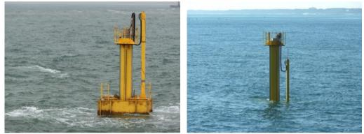
Figure 17. Test WEC at the coastal zone in Oarai port, floating (left) and sinking (right).
