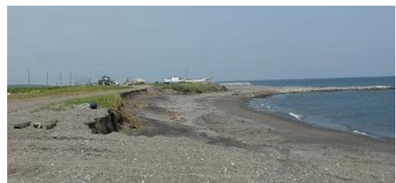
Figure 3. Eroded beach and vegetation down-drift of groin along line E-E in Figures 1 and 2.
