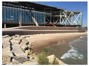
Figure 2 - Installed Wave Wall
