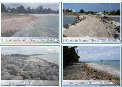
Nourishment site on the lagoon side (low wave energy). The openocean side appears to be protected by a seawall (more strongly)
