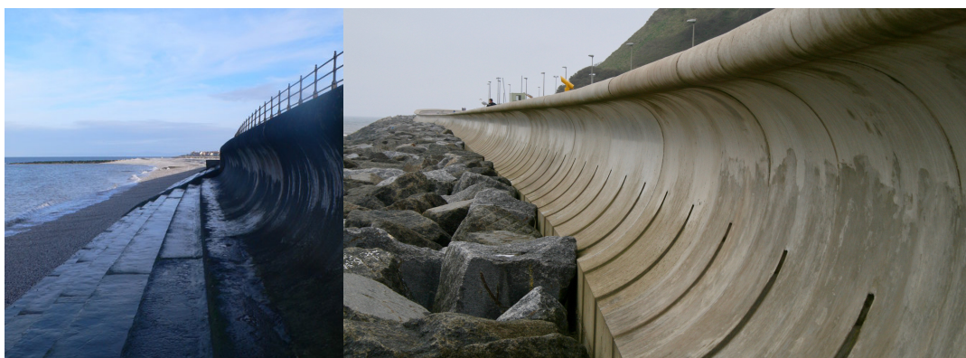
Figure 1. Wave return wall located in Penrhyn Bay, Great Britain reported in the left panel. Recurved seawall with rock armour at Scarborough reported in the right panel.
