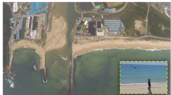
Figure. 3. - Field Investigation using Drone
