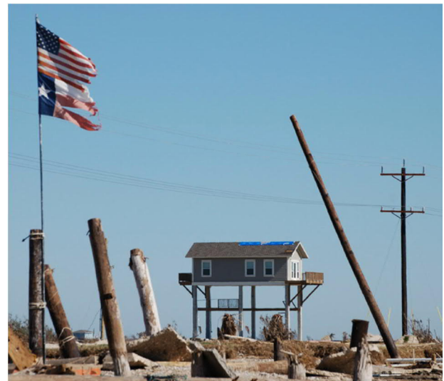
Figure 1 - Bolivar Peninsula, Texas after Hurricane Ike
