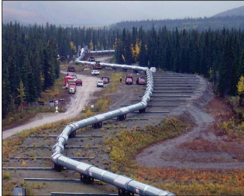
The Trans-Alaska Oil Pipeline, is designed to move 20-ft laterally and 5-ft vertically.
