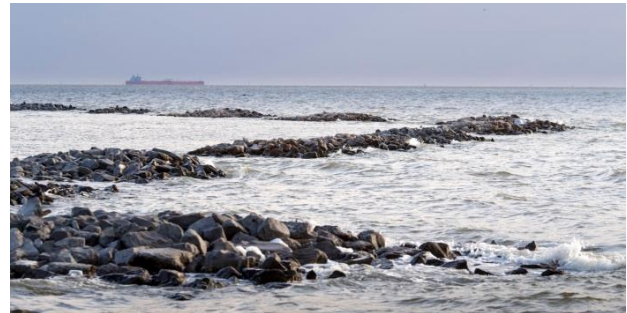
Figure 1 - Virginia Point Breakwaters
