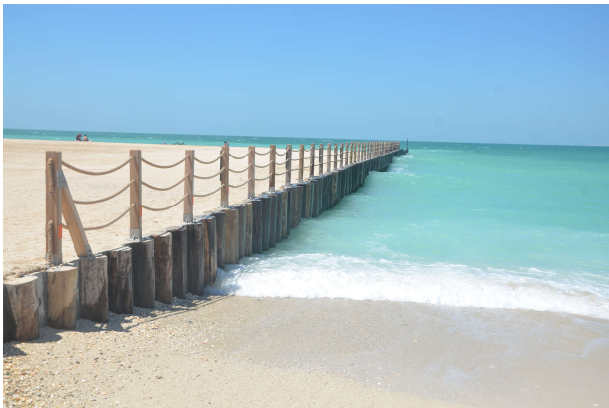
Figure 1 - Composite Groynes at Umm Suqeim Beach
