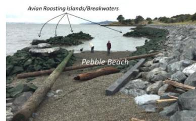
Figure 3 - Constructed pebble pocket beach, groin and roosting island breakwaters.
