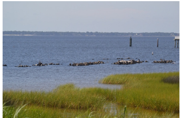
Figure 1 - This project in Pensacola, FL uses NNBF (oyster reefs offshore and fringing wetlands) for habitat enhancement and also protects a coastal roadway.
